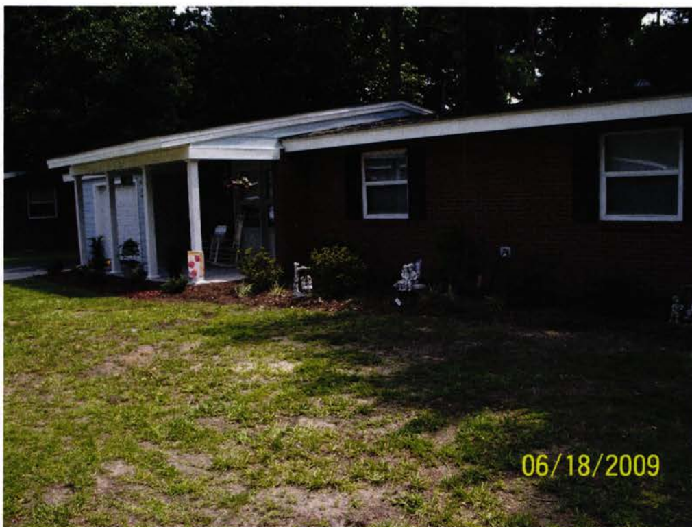
Picture 1: UST 1126Iris's location prior to excavation.
